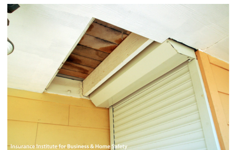
A horizontal enclosure, such as that shown here, can result in moisture-related degradation of wood and metal fasteners when deck boards are used.
