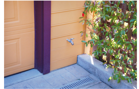
A noncombustible lower course of siding was used in this installation with otherwise combustible siding used in the higher courses. Source: Stephen L. Quarles
