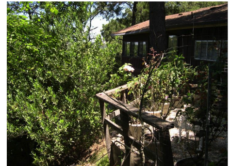
The defensible space on this property could be improved by removing vegetation to minimize the opportunity for fire to burn directly to the home. Source: Stephen L. Quarles
