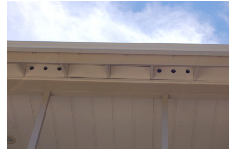
Gaps between the blocking and framing in the unvented truss bays would allow ember entry into the attic space. A sealant could be used to close gap. Source: Stephen L. Quarles
