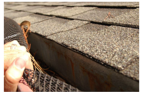
Gutter with integrated drip edge. Source: firecenter.berkeley.edu/bwmg/gutters.html
