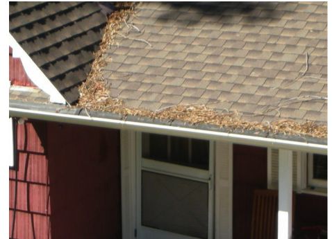
Debris accumulation on roof covering behind gutter cover device. Source: firecenter.berkeley.edu/bwmg/gutters.html
