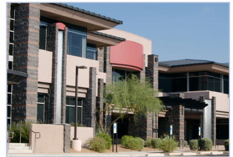
Vegetation too close to windows.
