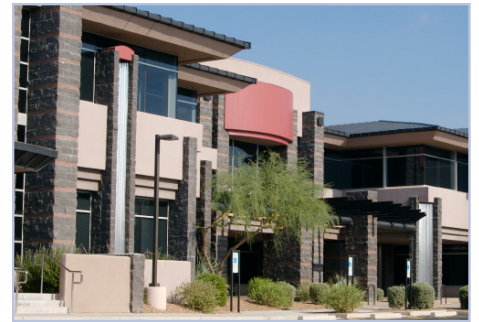
Vegetation too close to windows.
