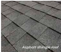
Asphalt shingle roof
