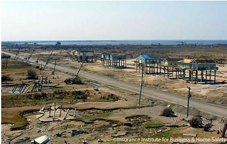
Figure 3: Homes on the Bolivar Peninsula following Hurricane Ike (2008). These structures were elevated above the 100-year flood level and built to the IBHS Fortified standard.
