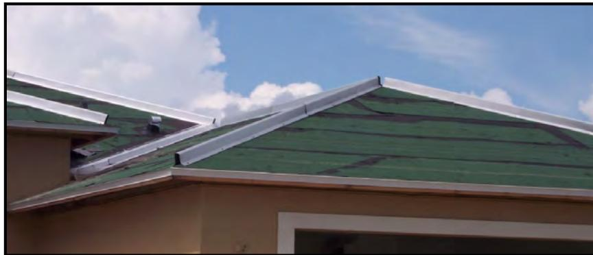
**Figure 3-3: Metal hat section alternative to nailer boards. Source: IBHS**
