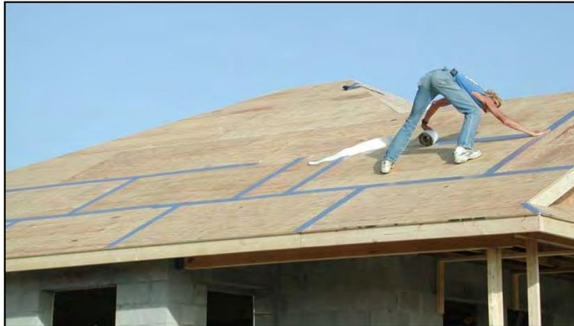
**Figure 3-3: Installation of sealed roof deck using self-adhering strips. Source: IBHS**
